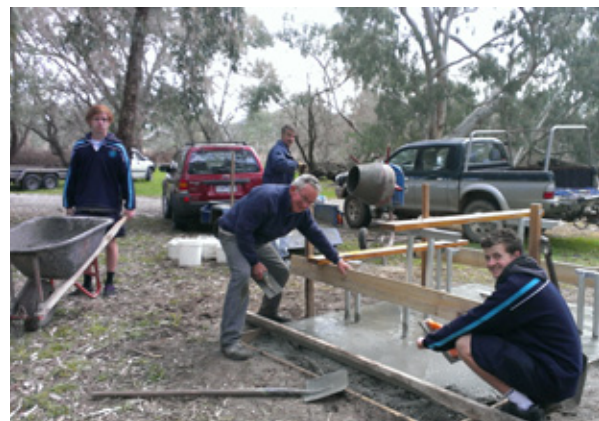
Wodonga Senior Secondary College students installing picnic tables they fabricated as part of their VCAL studies with materials donated by the Bonegilla Rail Trail Advisory Group.
